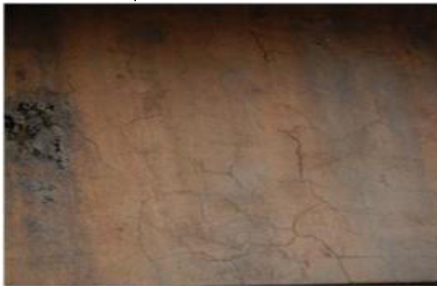
Figure 3-11: Pattern or Map Cracks
