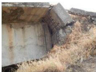
Deformation of Dirt Wall
