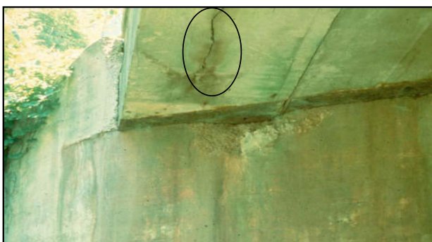
Figure 4-52: Longitudinal Cracks in Bottom Flange
