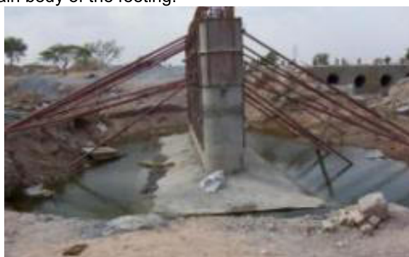
Figure 7-28: Reinforced Concrete Open Foundation
