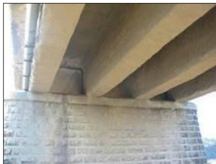
Figure 4-10: T-beam and Slab Bridge without Diaphragm
