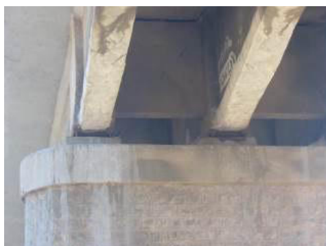
Figure 4-11: End Diaphragm not integrated into Deck Slab
