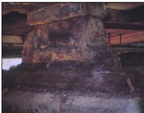
Figure 5-20: Heavy Corrosion of Steel Rocker Bearing
