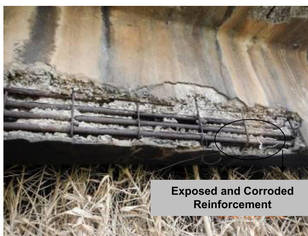
Figure 4-14: Exposed and Corroded Reinforcement
