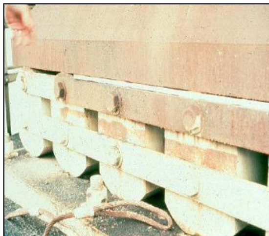
Figure 5-6: Segmental Rocker Nest Bearing
