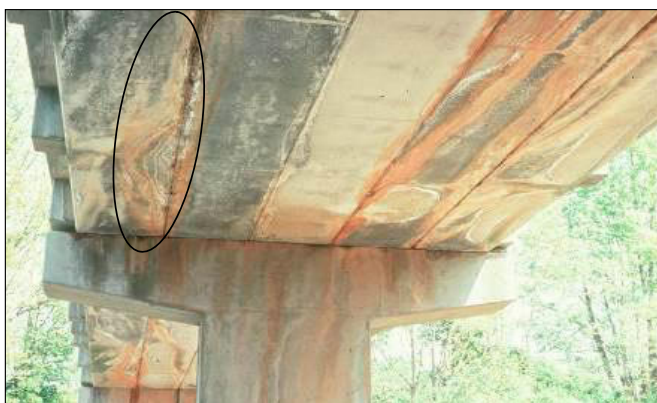
Figure 4-55: Joint Leakage and Rust Stain
