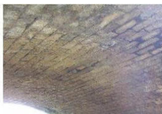
Loosening of Mortar Joints
