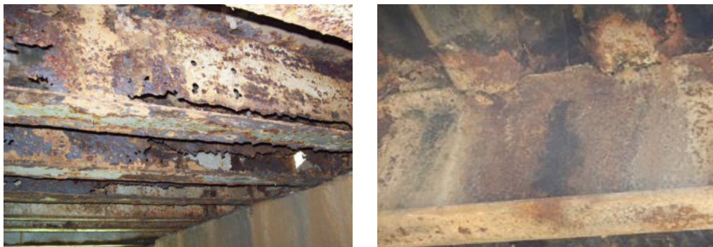
Figure 4-65: Schematic View of Corroded Steel Girder
