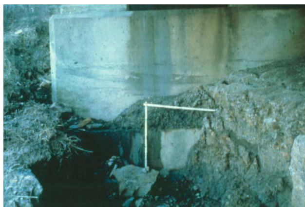
Figure 7-22: Erosion at Abutment Exposing Footing
