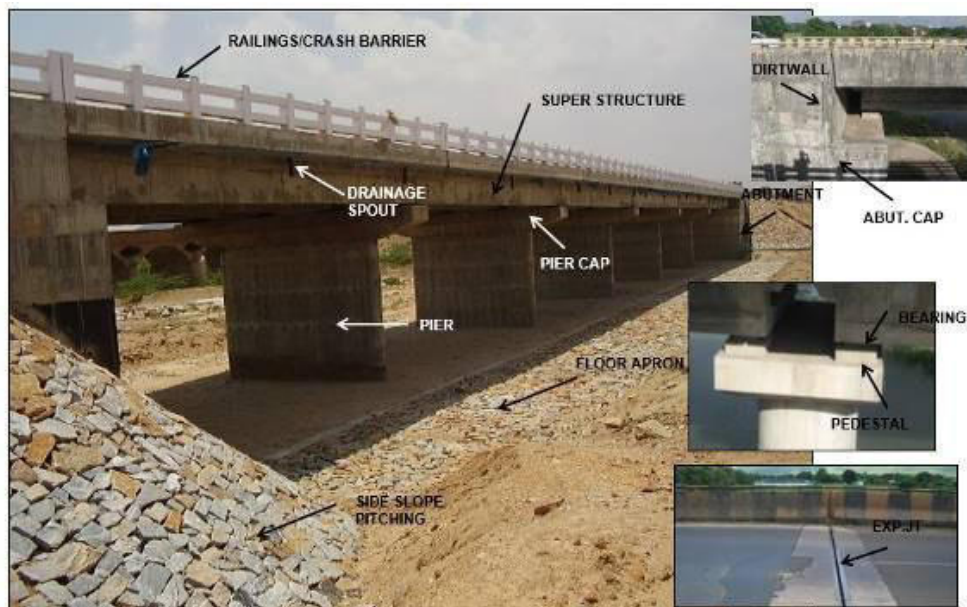
Figure 1-2: Various Components of Bridge
