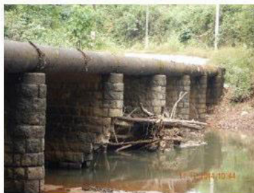
Cut Water / Pier Damaged due to Debris
