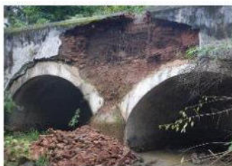
Spandrel wall Damaged
