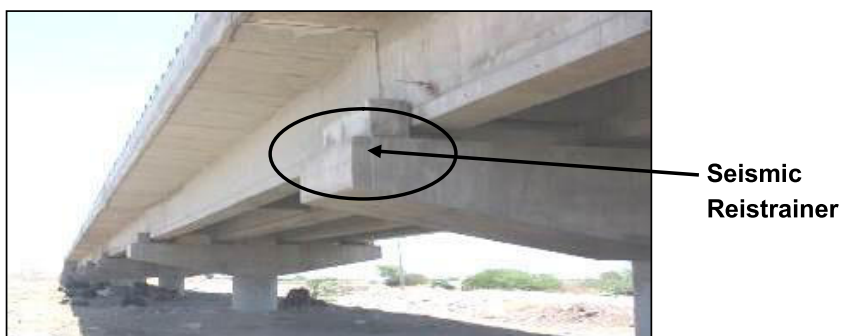
Figure 8-35: RCC Seismic Restrainer
