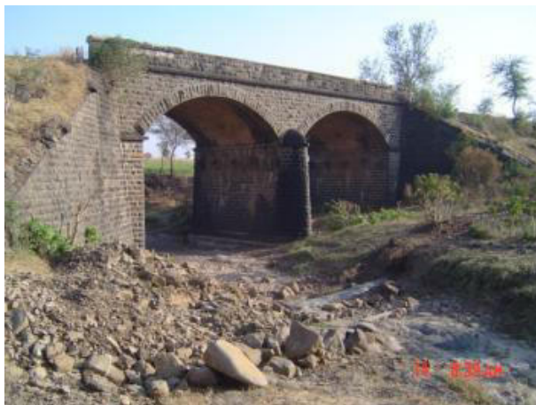
Figure 4-69: Elevation of a Stone Masonry Arch Bridge
