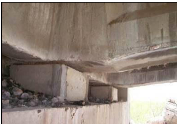
Figure 5-22: Accumulation of Debris at Bearing Pedestal Location
