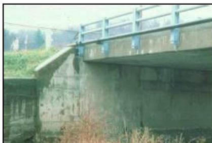
Figure 6-30: Integral Wing wall and MSE Wing wall
