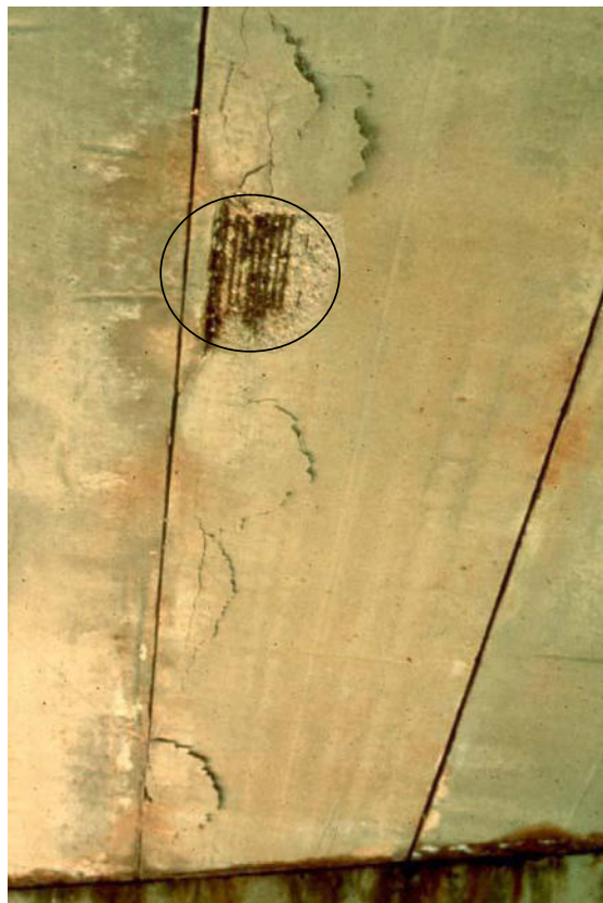
Figure 4-53: Spall and Exposed Reinforcement
