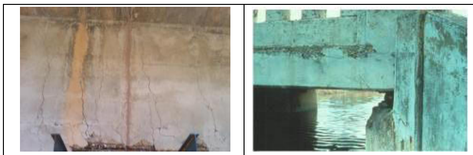
Figure 3-6: Flexural crack on T-Beam and Shear crack on Solid Slab
