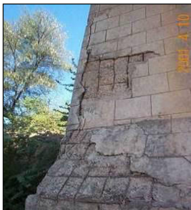
Figure 3-16: Exposed and Corroded Reinforcement in Sub Structure
