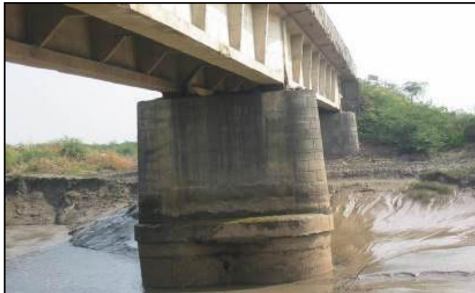
Figure 7-13: Local Scour at Pier Location
