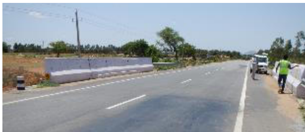
Figure 8-19: Reinforced Concrete New Jersey Type Crash Barrier
