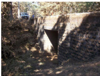
Figure 6-29: Masonry Wing Wall / Return Wall
