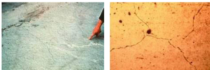
Figure 3-10: Temperature Cracks and Shrinkage Cracks
