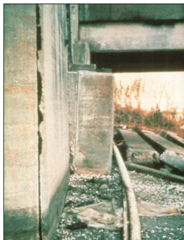
Figure 7-24: Rotational Movement at Abutment
