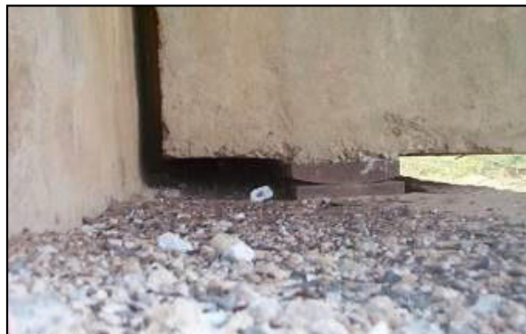
Figure 5-19: Movement of Sole Plate
