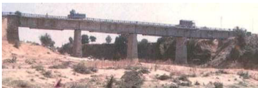
Figure 3-22: Concrete Superstructure on Brick Masonry Substructure
