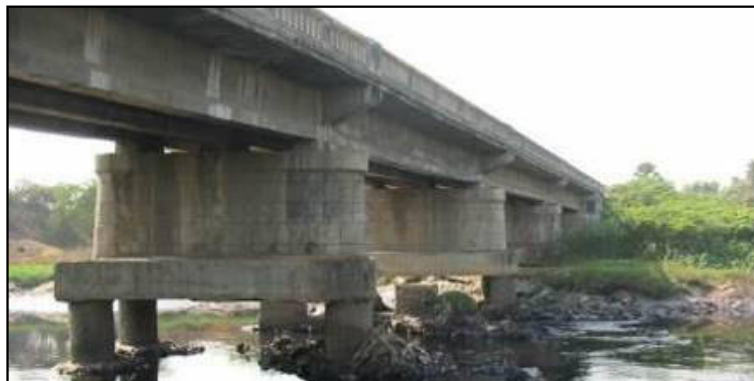
Figure 7-9: Increase in Scour due to Accumulation of Debris at Pier Location
