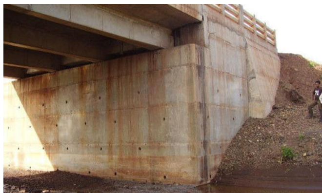
Figure 6-3: Solid Abutment
