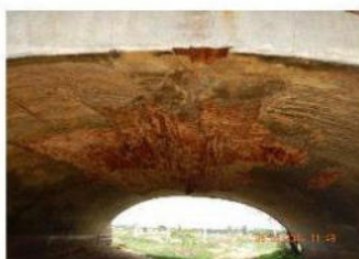
Severe loss of Bricks in Arch
