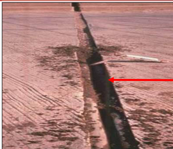
Figure 8-8: Dirt in a Seal Joint
