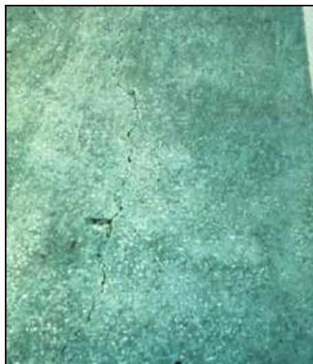
Figure 3-12: Longitudinal Cracks
