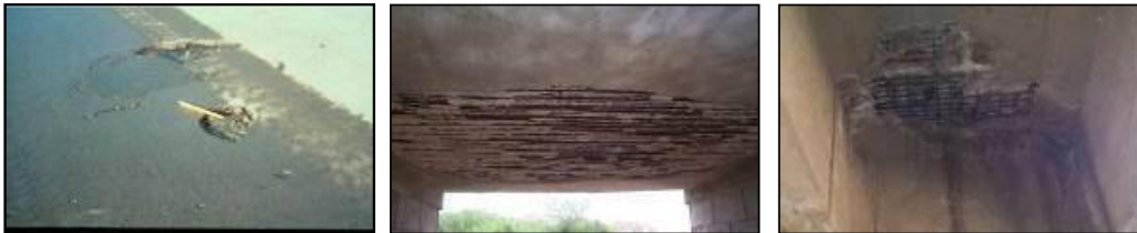
Figure 3-14: Small Spalling to Large spalling on a Concrete Deck
