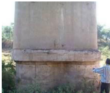
Figure 7-32: Scour Around Well Foundation
