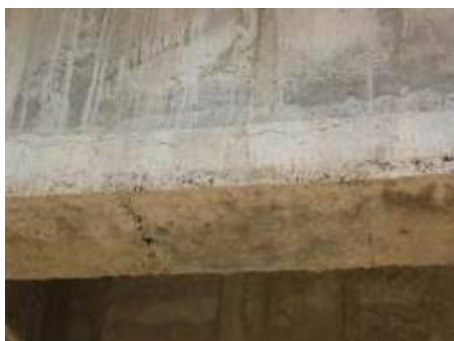
Figure 4-15: Longitudinal Crack at Girder Bulb
