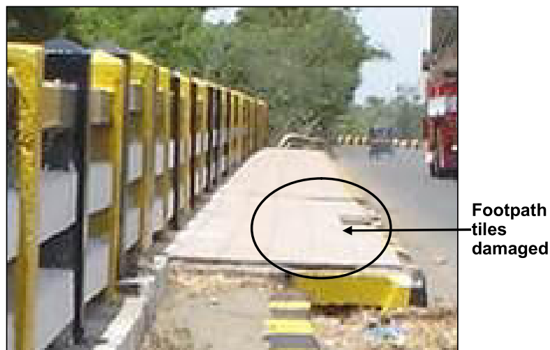
Figure 8-17: Footpath Tiles Damaged
