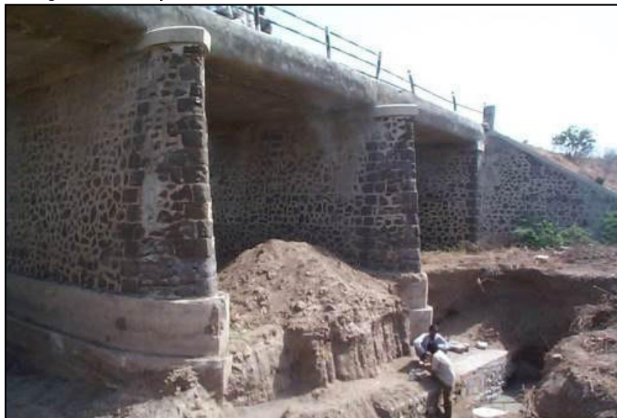
Figure 7-27: Masonry Open Foundation Partly Exposed
