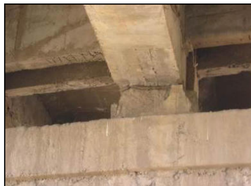
Figure 5-21: Cracks in Bearing Pedestal and Concrete Spalling in Pedestal
