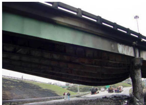
Figure 4-67: View of Bend due to severe heat Steel Girder
