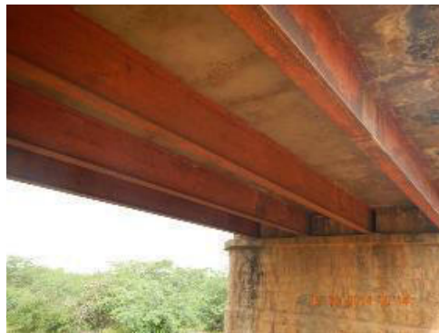
Figure 4-64: Schematic View of Steel I Girder
