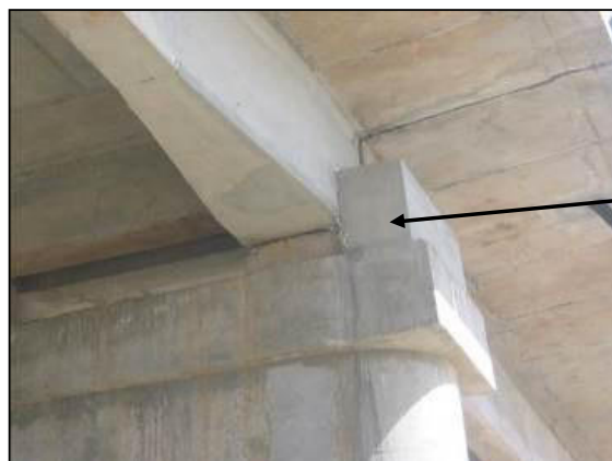
Figure 8-37: RCC Seismic Attachment on Pier Cap
