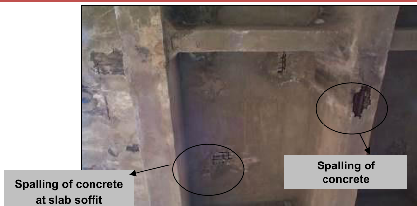
Figure 4-13: Cavity and Spalling of Concrete
