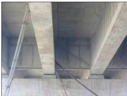
Figure 4-9: End Diaphragm Monolithic with Deck Slab
