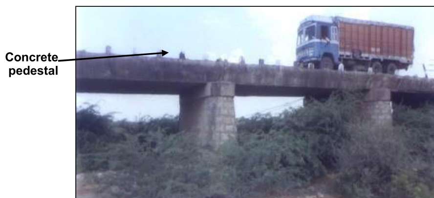
Figure 8-27: Steel Railings Pipe Missing
