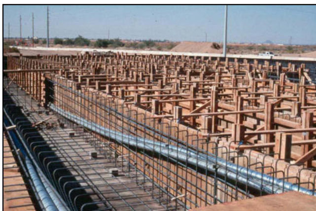
Figure 4-54: Post-tensioning Tendon Duct
