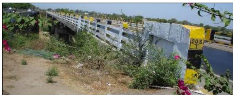
Figure 8-18: Reinforced Concrete Railing.
