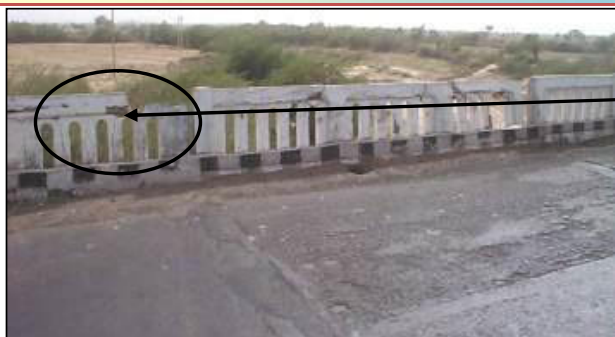
Figure 8-23: Broken and Damaged Railing
