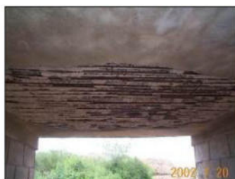
Spalling at Soffit of Slab
