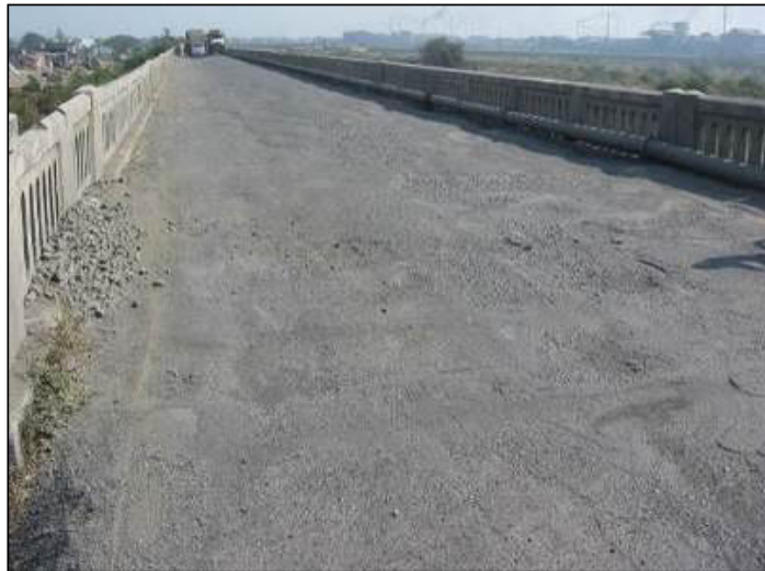
Figure 8-30: Damaged Wearing Coat
