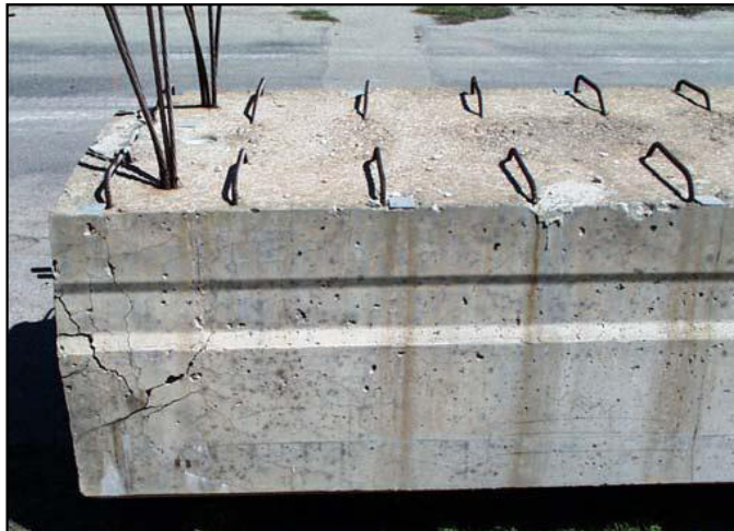
Figure 4-48: Spalled Concrete and Heavy Cracking
