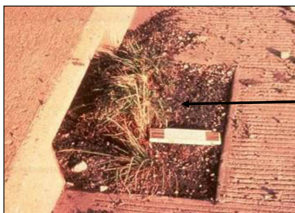
Figure 8-10: Clogged Drainage Inlet
