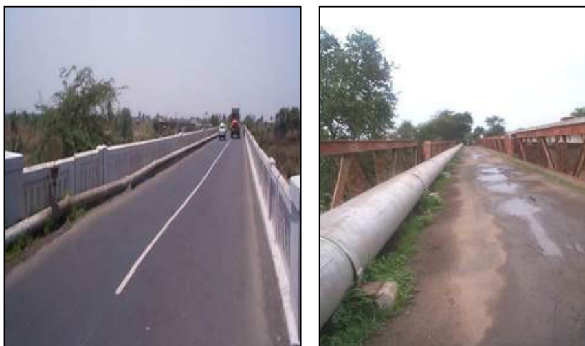
Figure 8-33: Service Line Over Bridge Deck inside the Carriageway
