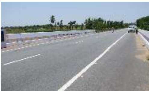
Figure 8-28: Bituminous and Concrete Wearing Coat
