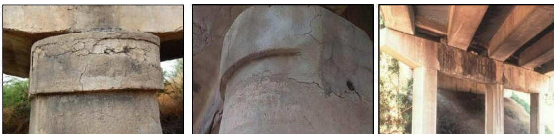
Figure 6-24: Cracks in Pier Cap
