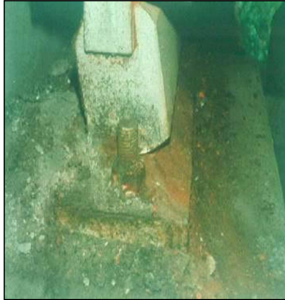
Figure 5-4: Segmental Rocker Bearing
