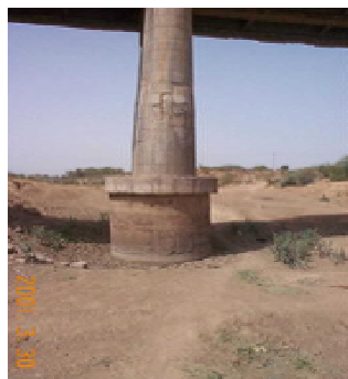
Figure 7-32: Scour Around Well Foundation
