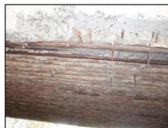
Reinf. Exposed and Corroded
