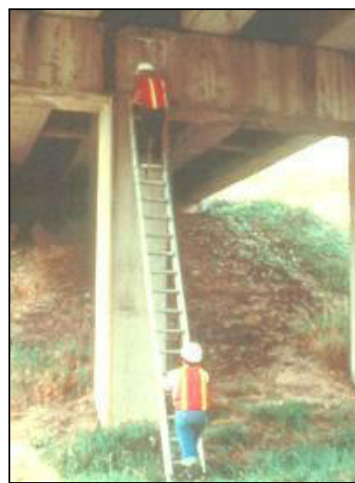
Figure 1-5: Inspection with the help of Ladder
