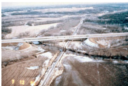
Wire Mesh and Grass Slope Stabilization
