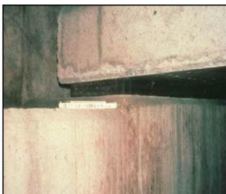
Figure 5-10: Elastomeric Bearing under a Girder and in Section
