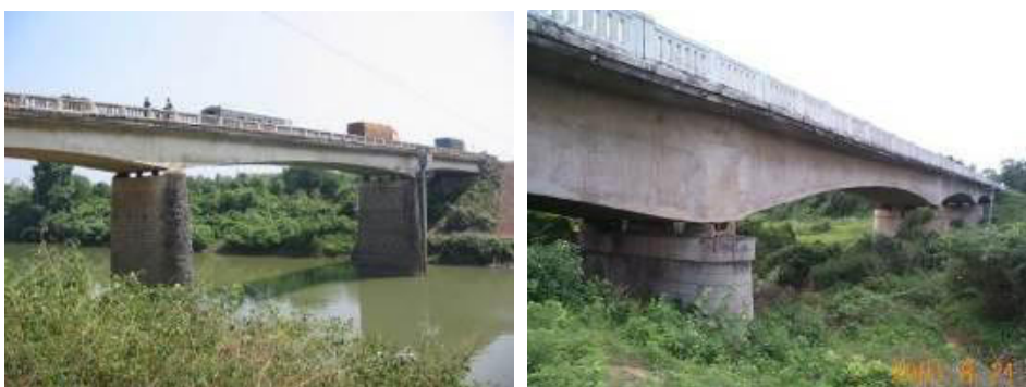
Figure 4-19: Typical Cast-in-place Concrete Box Girder Bridges
