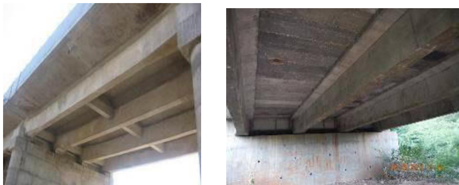
Figure 4-6: Simply-Supported T-beam and Slab Bridge of Constant Girder Depth
