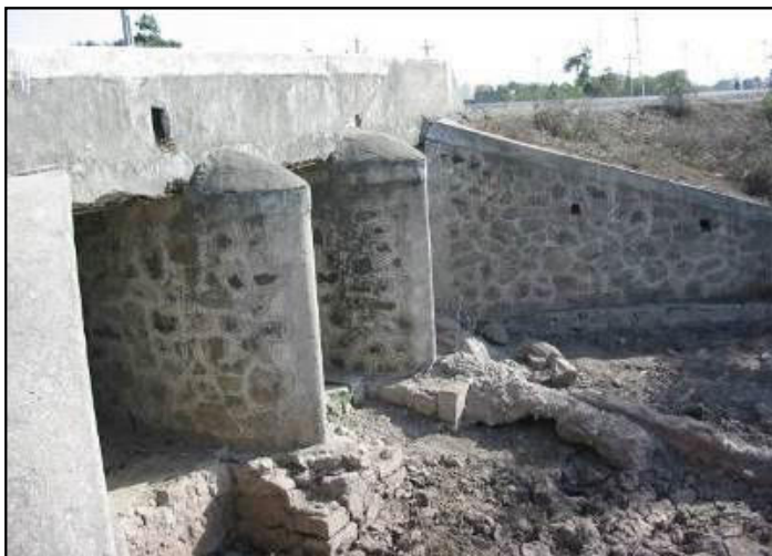
Figure 7-29: Damaged Masonry Open Foundation
