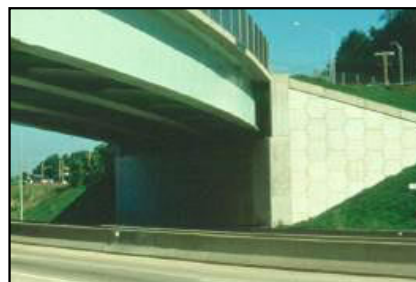
Figure 6-30: Integral Wing wall and MSE Wing wall
