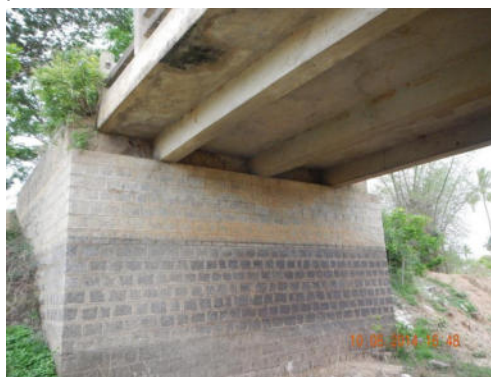
Stone Masonry Abutment
