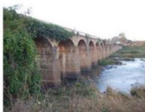
Vegetative Growth in Spandrel wall
