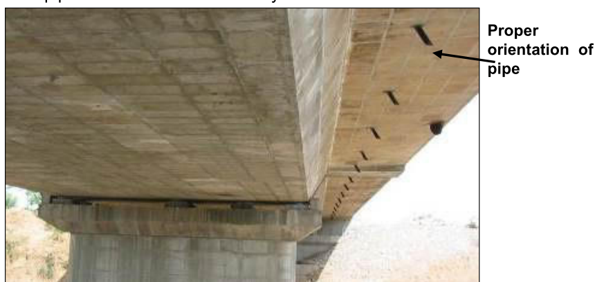
Figure 8-12: Proper Orientation of Drainage Pipe
