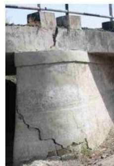
Crack in pier due to Settlement
