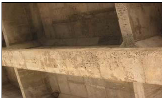
Figure 3-15: Honeycomb of Concrete
