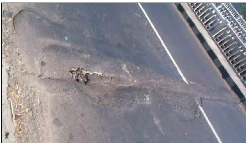
Figure 8-9: Damaged expansion joints
