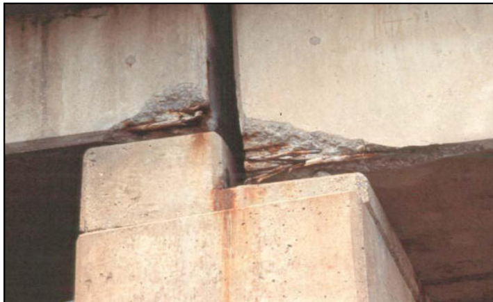
Figure 4-50: Spalled Ends
