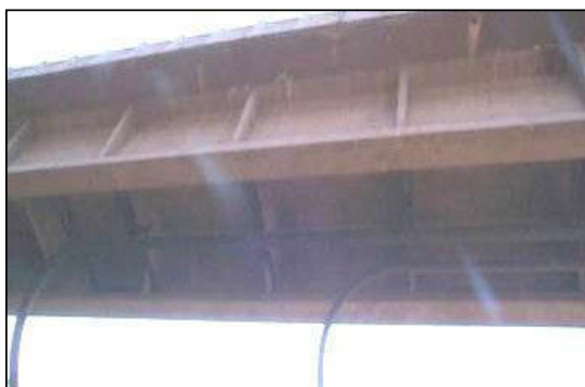
Figure 8-34: Partially Collapsed Service Lines
