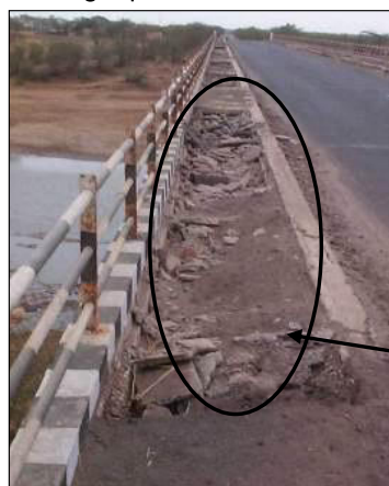
Figure 8-16: Broken Footpath
