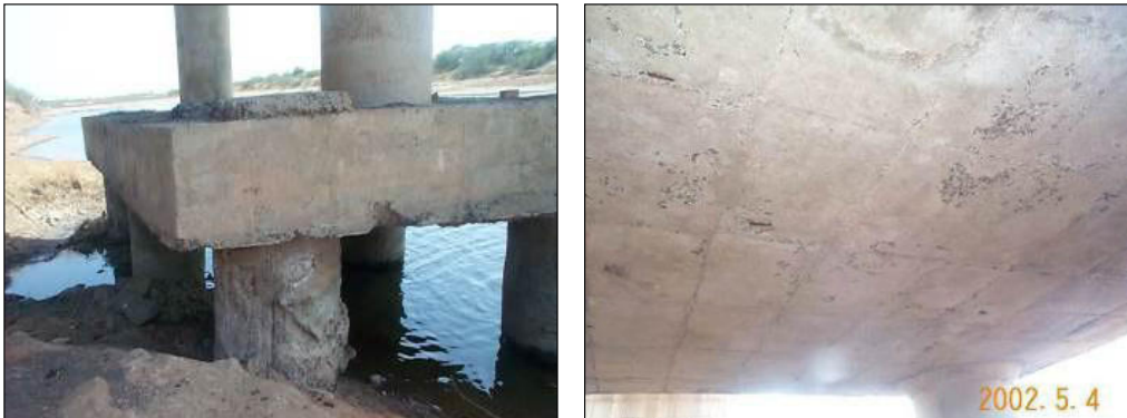
Figure 7-37: Erosion of Concrete Surface at Exposed Portion of Piles and Concrete Surface Defects at the Soffit of an Exposed Pile Cap
