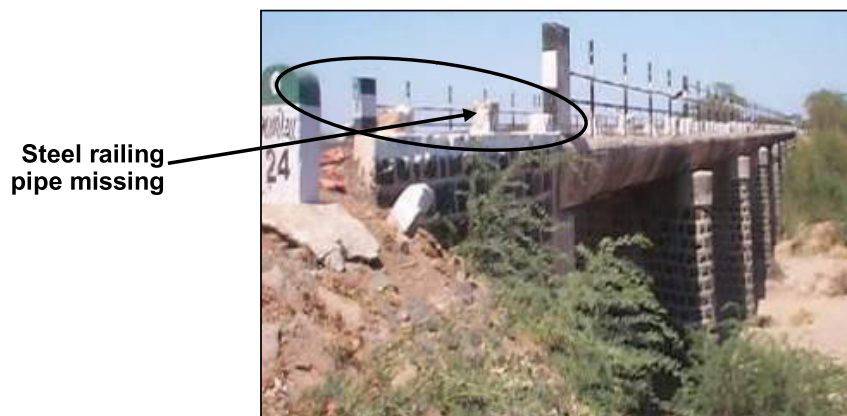
Figure 8-26: Pipe is missing from Steel Railing
