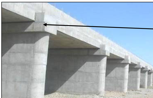
Figure 8-36: RCC Seismic Attachment on Pier Cap
