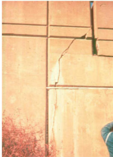
Figure 7-17: Cracks in Abutment due to Settlement
