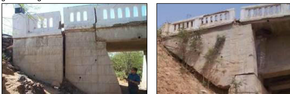
Figure 6-32: Dislodged Wing Wall
