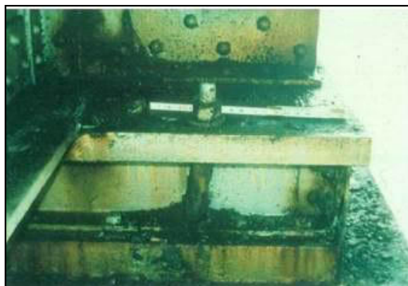
Figure 5-17: Damaged Anchor Bolt
