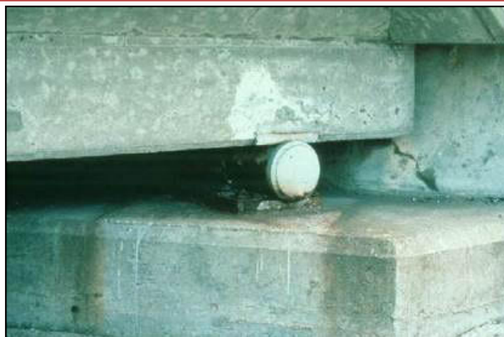
Figure 5-2: Single Roller Bearing
