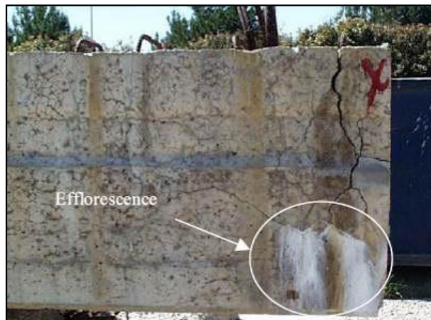
Figure 4-49: Efflorescence
