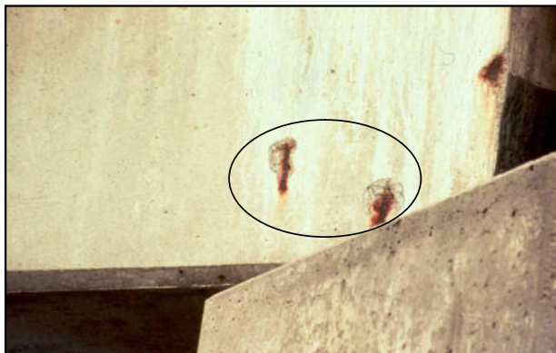
Figure 4-51: Exposed Bars at End of Box
