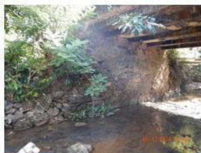
Poor Quality of Stones and workmanship
