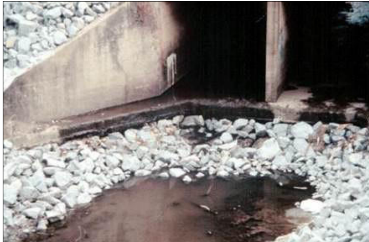
Figure 7-11: Failed Bed Protection Riprap due to Scour
