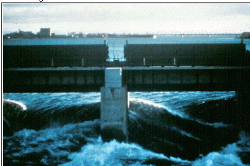
Figure 7-1: Flood Flow around a Pier Showing Stream Flow Velocity
