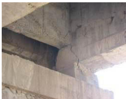
Figure 4-16: Bearing Crack
