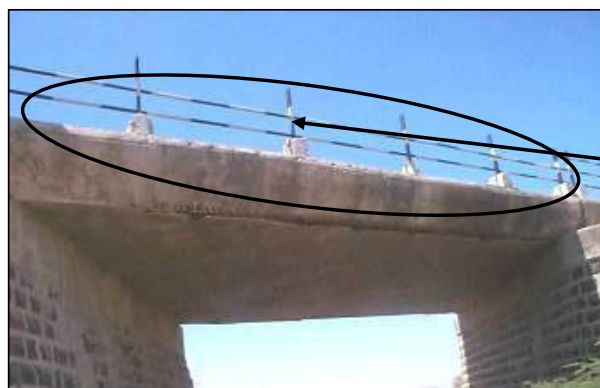
Figure 8-25: Missing Steel Pipe at top of Railing
