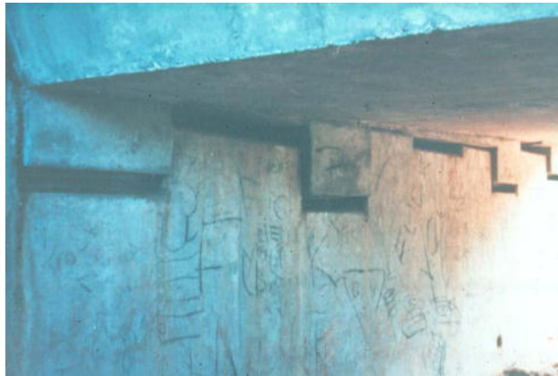
Figure 4-23: Shear Crack Location near an Abutment
