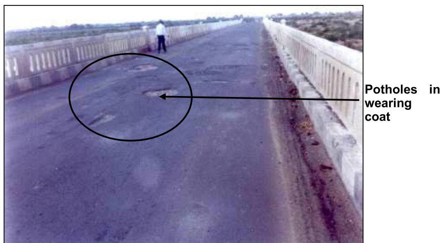
Figure 8-29: Pot Holes in Wearing Coat
