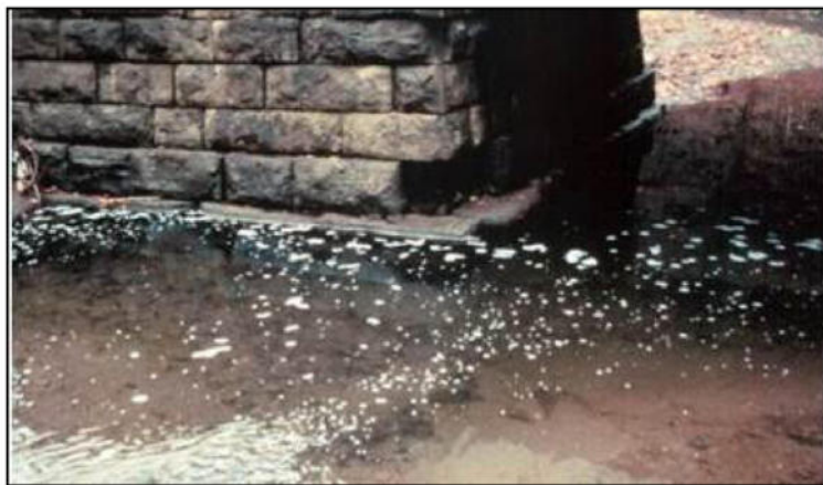
Figure 7-7: Local Scour at an Abutment
