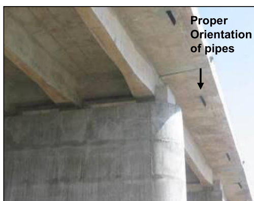
Figure 8-11: Proper Projected Length of Drainage Pipe and Missing Drainage Pipe
