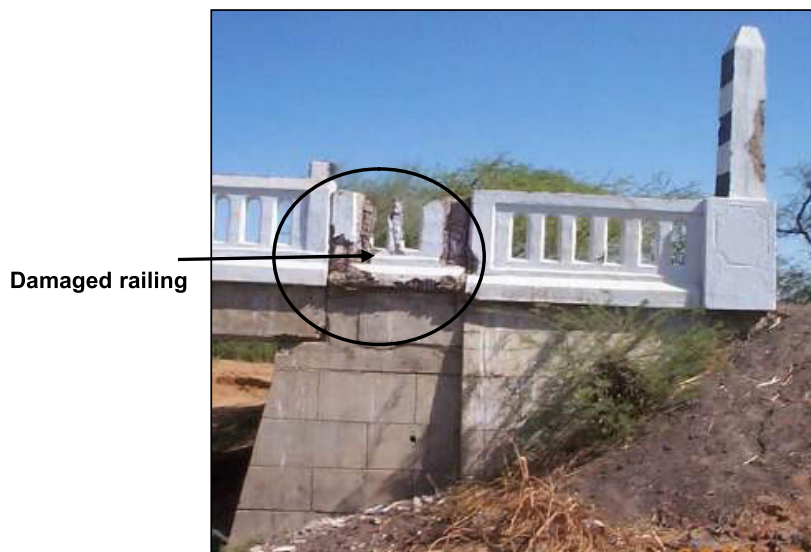
Figure 8-24: Damaged RCC Railing
