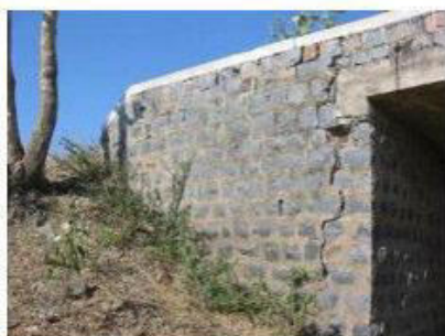
Cracks due to Earth Pressure
