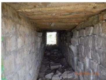
Damaged Stone Masonry due to Insufficient Mortar Joints
