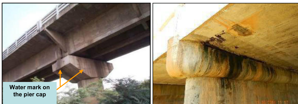
Figure 6-21: Water Marks on Pier Cap
