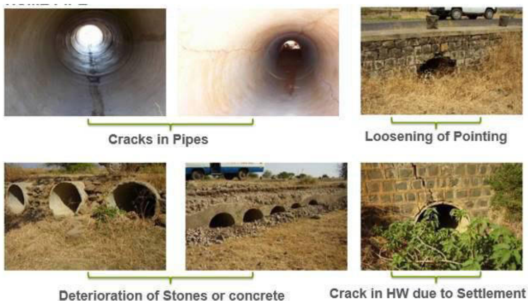
Figure 3-2: Showing Various condition of Pipe Structure
