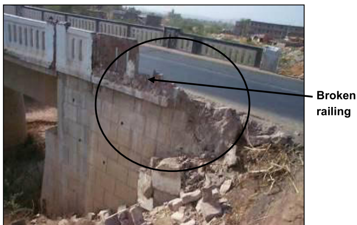
Figure 8-22: Broken Railing
