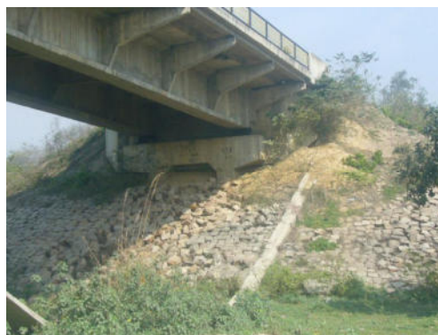
Figure 6-2: Spill through (Open) Abutment
