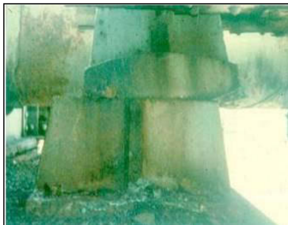
Figure 5-18: Frozen Rocker Bearing
