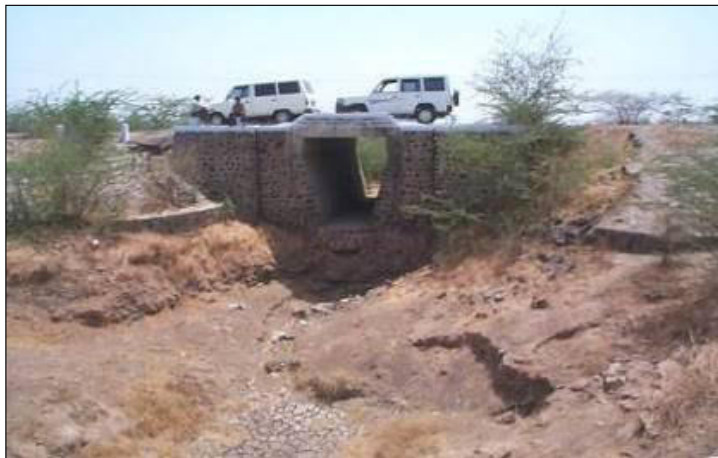
Figure 7-12: Excessive Scour in the Down Stream of a Slab Culvert (Bed Protection Entirely Washed Away and Embankment Damaged)
