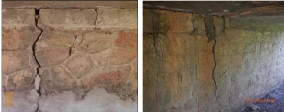
Figure 3-19: Cracks, Loss of Mortar at Joint in Masonry Substructure
