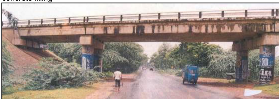
Figure 4-57: Voided Slab Super-Structure
