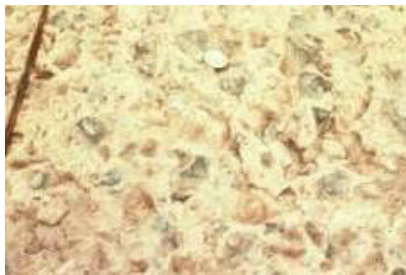
Figure 3-13: Various types of Scaling
