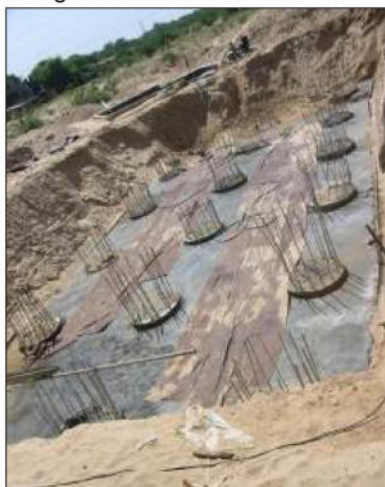
Figure 7-36: Pile Cap below GL and Pile Cap above Natural Ground Level
