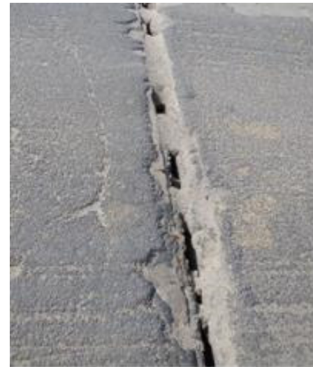
Damaged Expansion Joint
