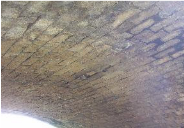
Loosening of Mortar Joints
