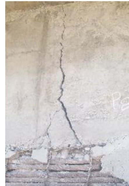
Severe Crack in Gir
