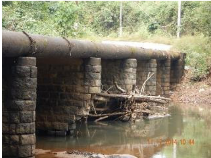
Cut Water / Pier Damaged due to Debris
