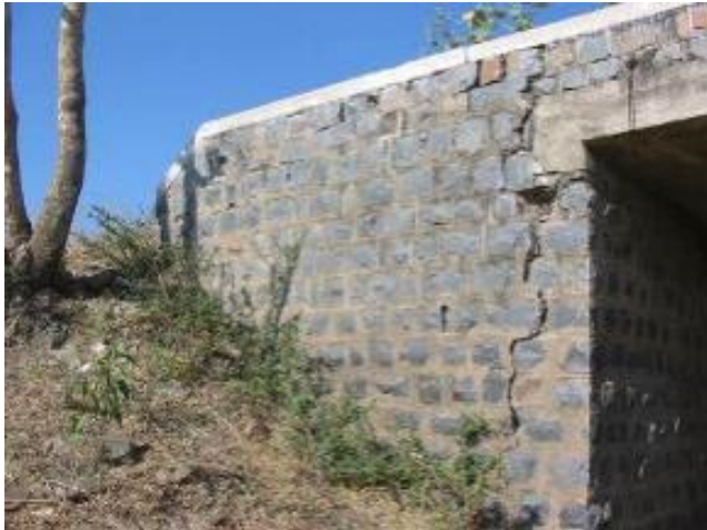
Cracks due to Earth Pressure
