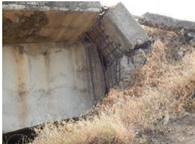
Deformation of Dirt Wall
