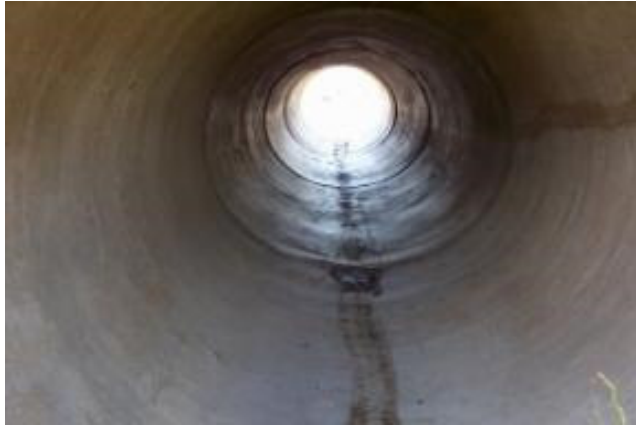
Cracks in Pipes
