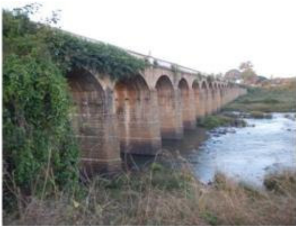
Vegetative Growth in Spandrel wall
