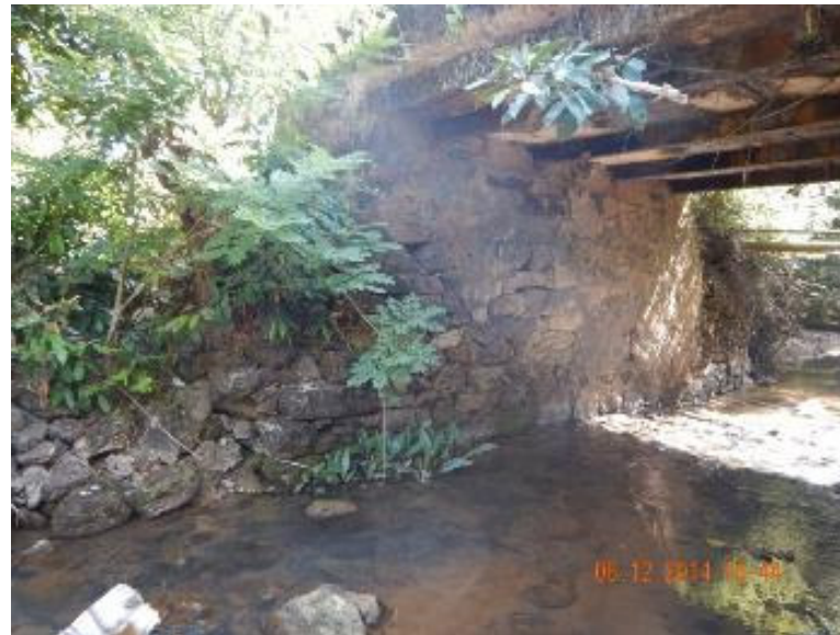
Poor Quality of Stones and workmanship
