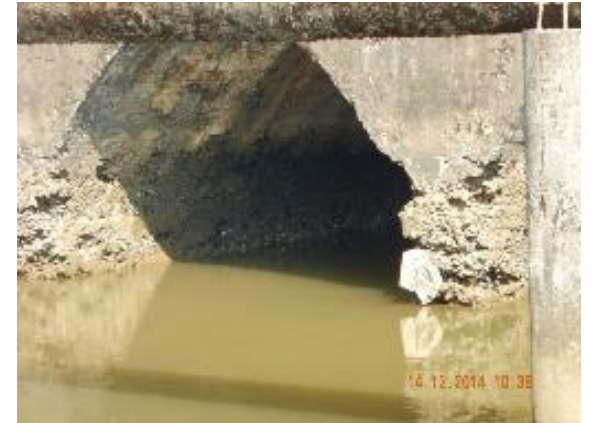
Poor Concrete in Pipes
