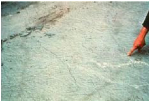
Temperature Cracks
