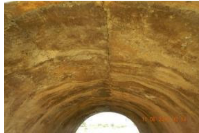
Minor Cracks in Pipes
