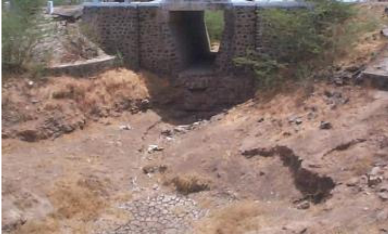
Excessive Scour on D/S Side of Structure
