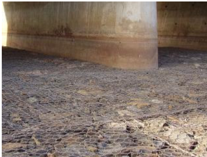
Gabions and Mattresses for Floor Protection
