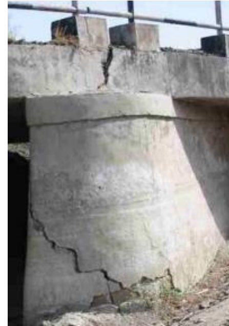
Crack in pier due to Settlement
