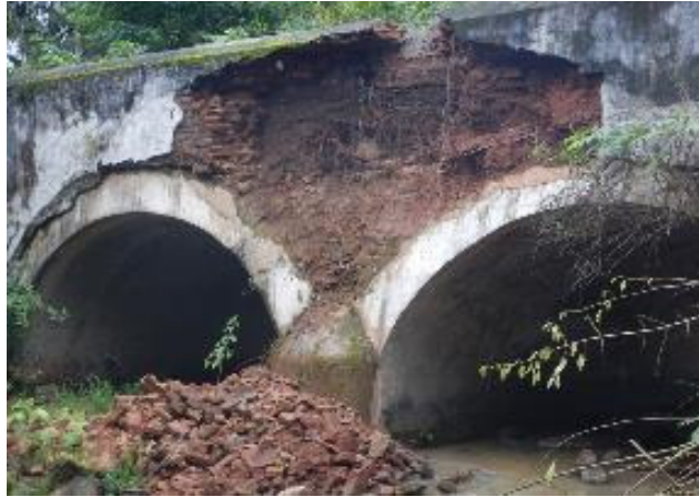
Spandrel wall Damaged
