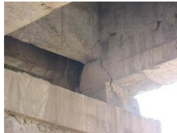
Bearing Crack
