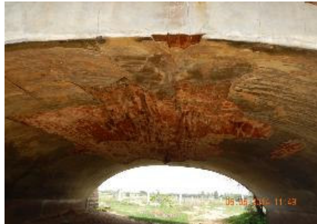
Severe loss of Bricks in Arch
