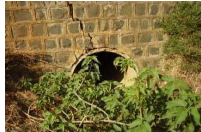
Crack in HW due to Settlement
