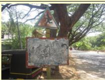
**CLEAR** – the shape and colour of the sign, as well as the legend/symbol, have to be able to be read from a sufficient distance. This warning sign is not clear and should be replaced.
