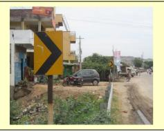
**GUIDE.** If the geometry of the design cannot be improved, one option is to install chevron alignment markers to guide drivers through tight curves. Strong edge lines also assist.
