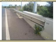
This photo shows W beam barrier firmly attached to a bridge; the posts become more closely spaced to add strength to the barrier close to the rigid abutment.
